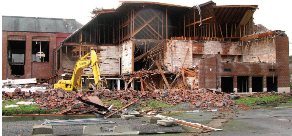
The demolition of Washington Grade School took place in February 2013.
