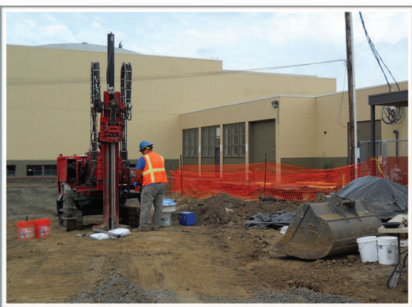
Collecting environmental samples with a drill rig
