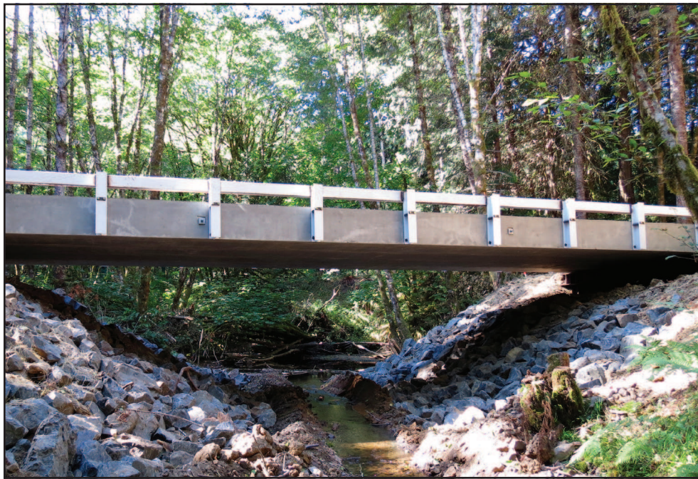
A new bridge built by Siegmund Construction on Pebble Creek.
