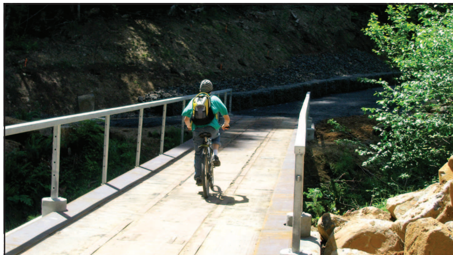
A bike rider using the new bridge at the Alder Creek crossing.
