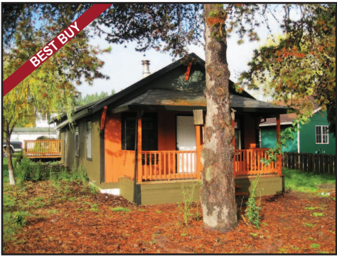
1107 Ruth Avenue..... $79,900 BEST PRICED restored stickbuilt home out of the flood plain. Low property taxes! 3bd/2ba, 1192sq.ft!
