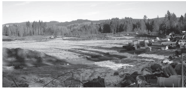
The school construction site in Vernonia on January 3, 2011.
