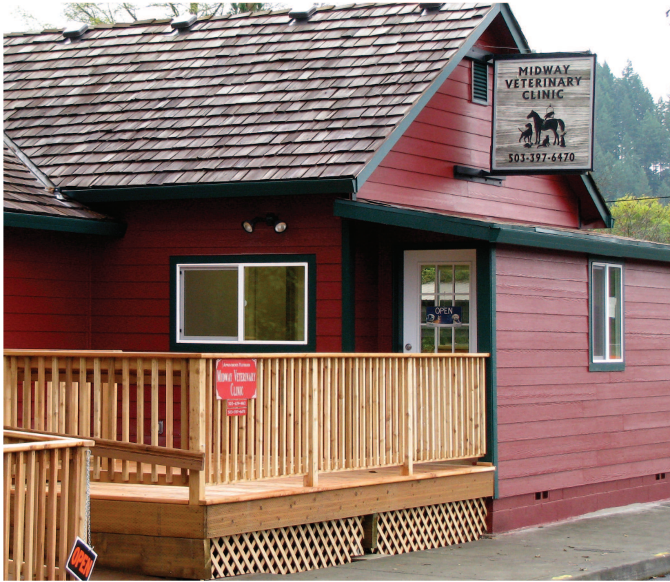
Midway Vet has moved from their Bridge Street location to their newly renovated office at 700 Weed Avenue. They will be hosting an open house on Sunday, November 21st from 12 to 3 PM. Everyone is invited to stop by for a tour of the new facility, coffee and snacks and lots of free pet gifts.
