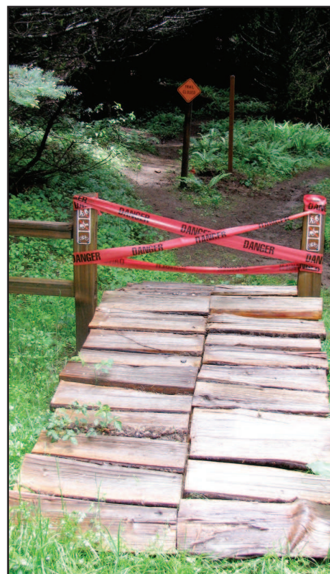
This Roll-over ramp will be the entrance to the mountain bike trail area at Stub Stewart State Park.
