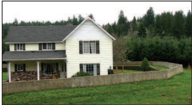
Bill Sword has built a four-foot high concrete wall around his property in Vernonia.
