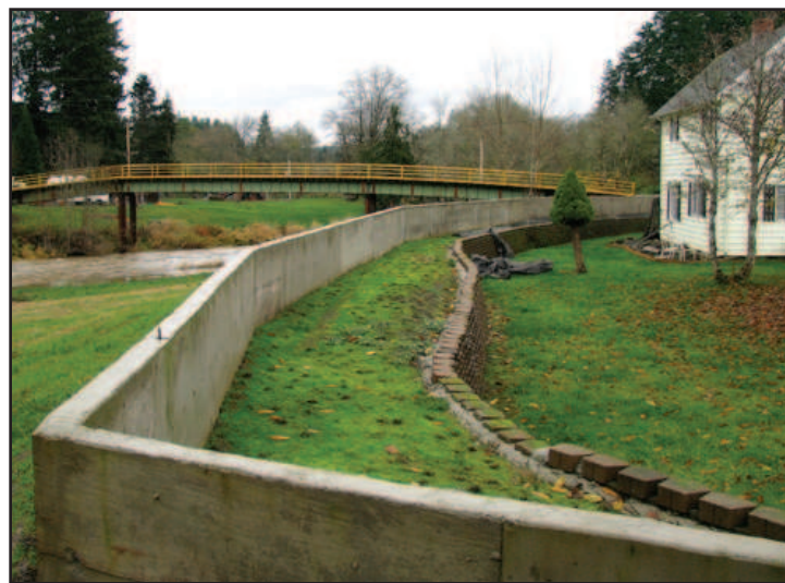
After the 1996 flood Bill Sword built a dirt berm around his house and shop to keep flood waters out. You can see that initial berm here, and the new higher wall Sword added when waters came over the berm in 2007.
