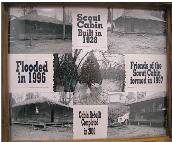
Shirlee Daughtry created a history of the Scout Cabin Renovation, that is framed in one of the old windows (above). Here is a look at the original building before local residents rebuilt the cabin.
