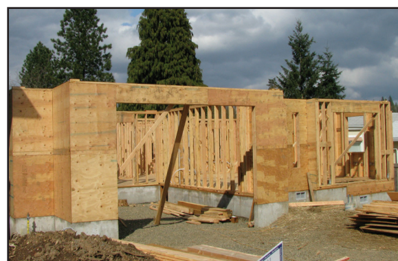
Christian Aid Ministries Workers helped frame the home being built for Dean and Kendra Schaumburg.
