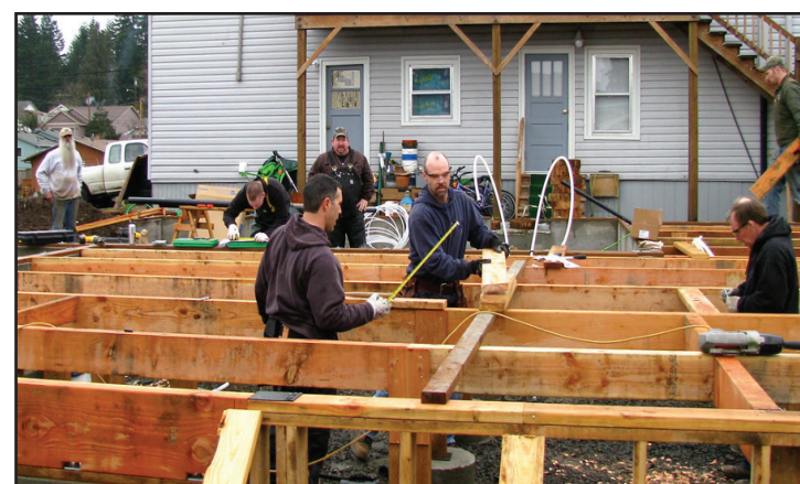
Plumbers and Pipe Fitters Local 290 donate time to help with the Schaumburg House.
