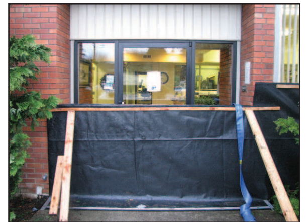
WOEC tries blocking doorways to keep water out
