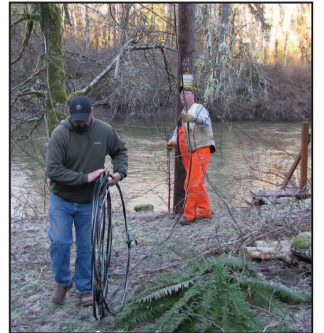
Randy Heath and Jim King reconnect power to a WOEC customer.
