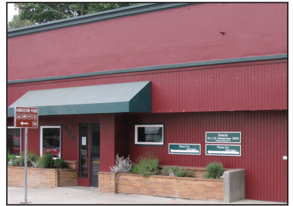
The Rock Creek Professional Building has a new look.
