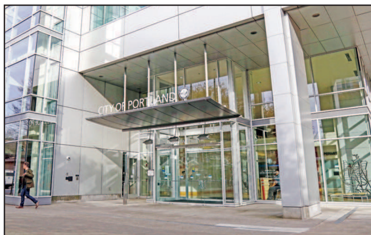
Thanks to permit fees paid by the construction industry, the Bureau of Development Services paid off the bond last year on its office building at 1900 SW Fourth Ave. Then the city raised its rent to $45.50/sq ft./year.
