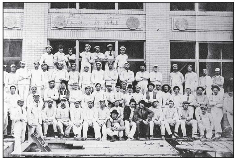
A plastering crew in 1912 breaks to pose for a photo in front of the Multnomah Hotel. The hotel, now an Embassy Suites, is still at SW Third and Pine.
