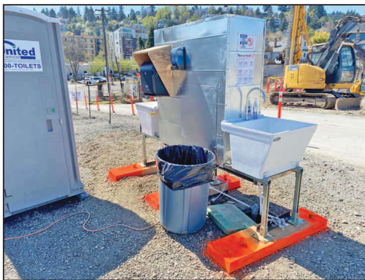
STRANGE NEW CONSTRUCTION EQUIPMENT: Because construction sites typically lack running water for hand-washing, Hoffman Construction is constructing and setting up its own hand-washing stations.
