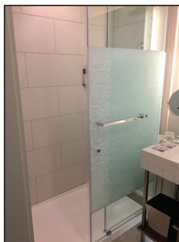
In 600 rooms at the Hyatt Regency, shower tiles were set by a non-union company that violated prevailing wage and other laws.
