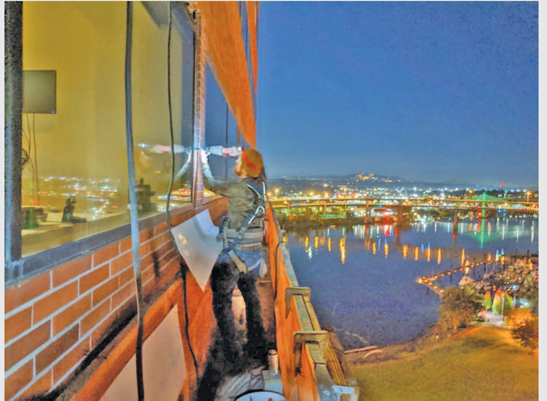
Near midnight near the top of Portland's 18-story Umpqua Bank Plaza building, Bricklayers Local 1 apprentice Henry Davidson IV uses a rotary hammer with a light attached to waterproof a window for Pioneer Waterproofing. The work takes place at night so tenants aren't interrupted by the noise. On a clear night in mid-October, the views are spectacular. (Photo by journeyman coworker Jeremy McCarty.)
