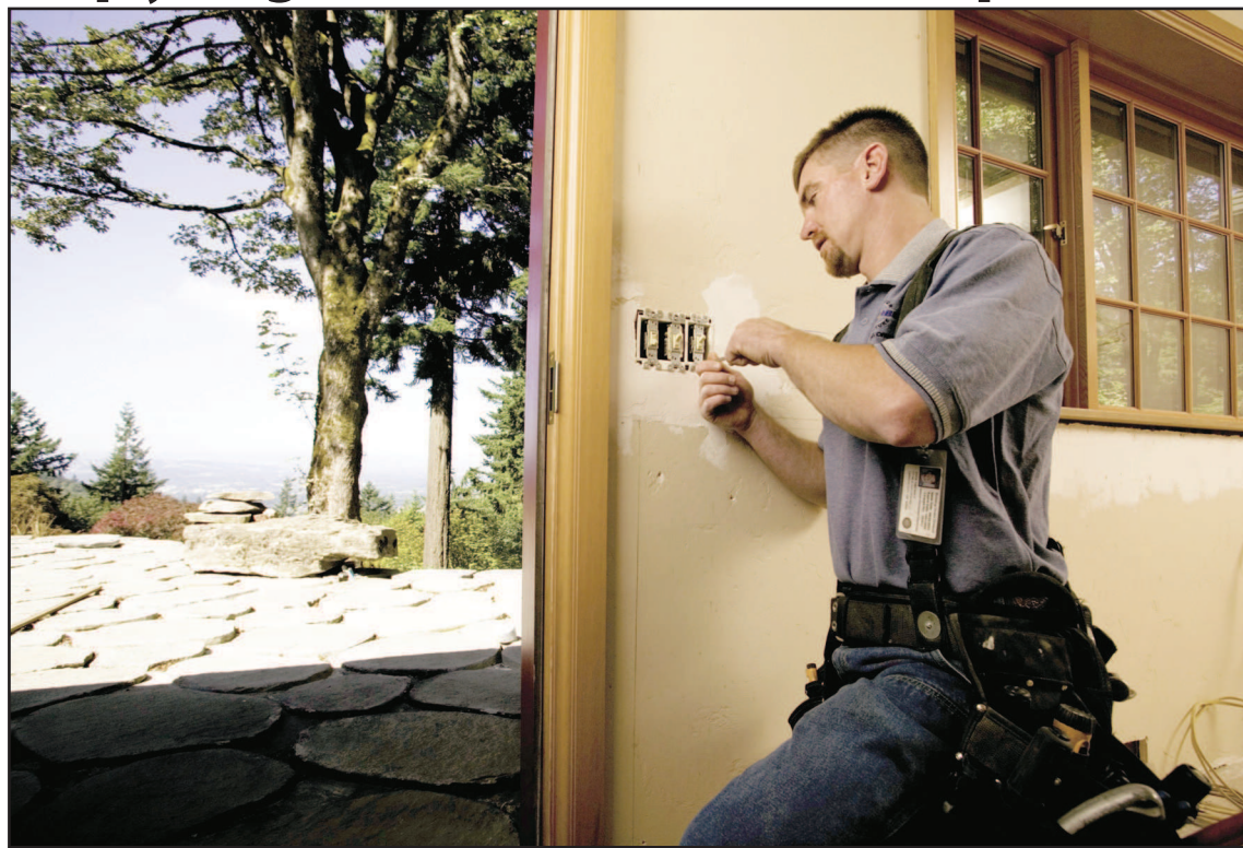
HOME IMPROVEMENT: IBEW Local 48 member Timothy Dyck on the job.
