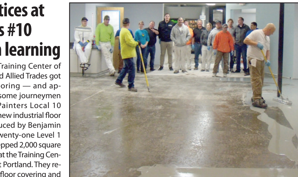
ABOVE: Jeff Spillane of Benjamin Moore & Co. (right) shows members of Painters Local 10 how to apply a 100 percent solids coating to the Regional Training Center floor. Journeyman Raymond Stallworth (left) helps out. BELOW: Apprentice Shannon Starr (left), and Hailey Suydam of Dicks color center use spiked shoes to apply a thick Industrial coating to the floor. Experts from Benjamin Moore & Co. teamed with the Regional Training Center to teach apprentices the latest in industrial coating products.
