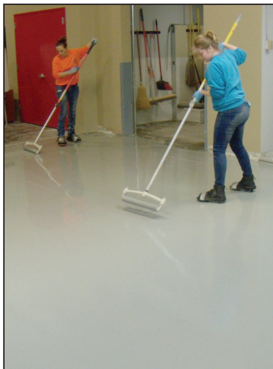
ABOVE: Jeff Spillane of Benjamin Moore & Co. (right) shows members of Painters Local 10 how to apply a 100 percent solids coating to the Regional Training Center floor. Journeyman Raymond Stallworth (left) helps out. BELOW: Apprentice Shannon Starr (left), and Hailey Suydam of Dicks color center use spiked shoes to apply a thick Industrial coating to the floor. Experts from Benjamin Moore & Co. teamed with the Regional Training Center to teach apprentices the latest in industrial coating products.
