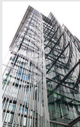
A green retrofit of the Portland federal building was one of just a few local ARRA projects that created jobs.
