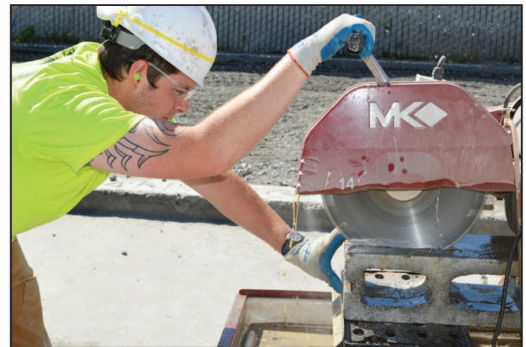
WHAT'S MISSING FROM THESE PICTURES? DUST. Bricklayers Local 1 apprentice Krista Kiser, above, grinds a mortar joint with a vacuum attached. Below, her fellow apprentice Tristan Burke operates a brick saw with a water hose attachment. On Page 1, apprentice Robert Griggs operates the same brick saw without the water — generating the dust that causes silicosis.
