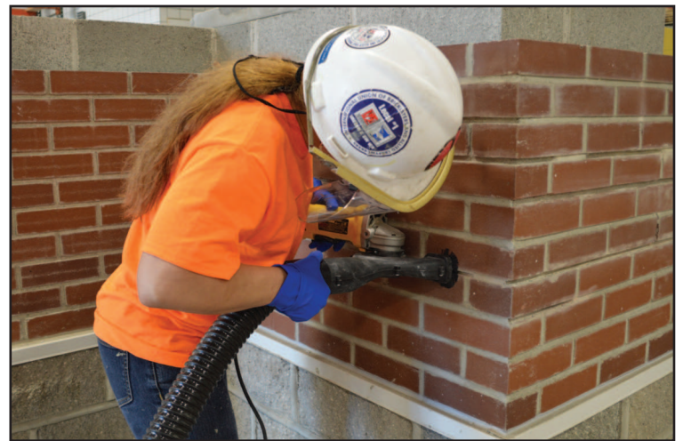
WHAT'S MISSING FROM THESE PICTURES? DUST. Bricklayers Local 1 apprentice Krista Kiser, above, grinds a mortar joint with a vacuum attached. Below, her fellow apprentice Tristan Burke operates a brick saw with a water hose attachment. On Page 1, apprentice Robert Griggs operates the same brick saw without the water — generating the dust that causes silicosis.
