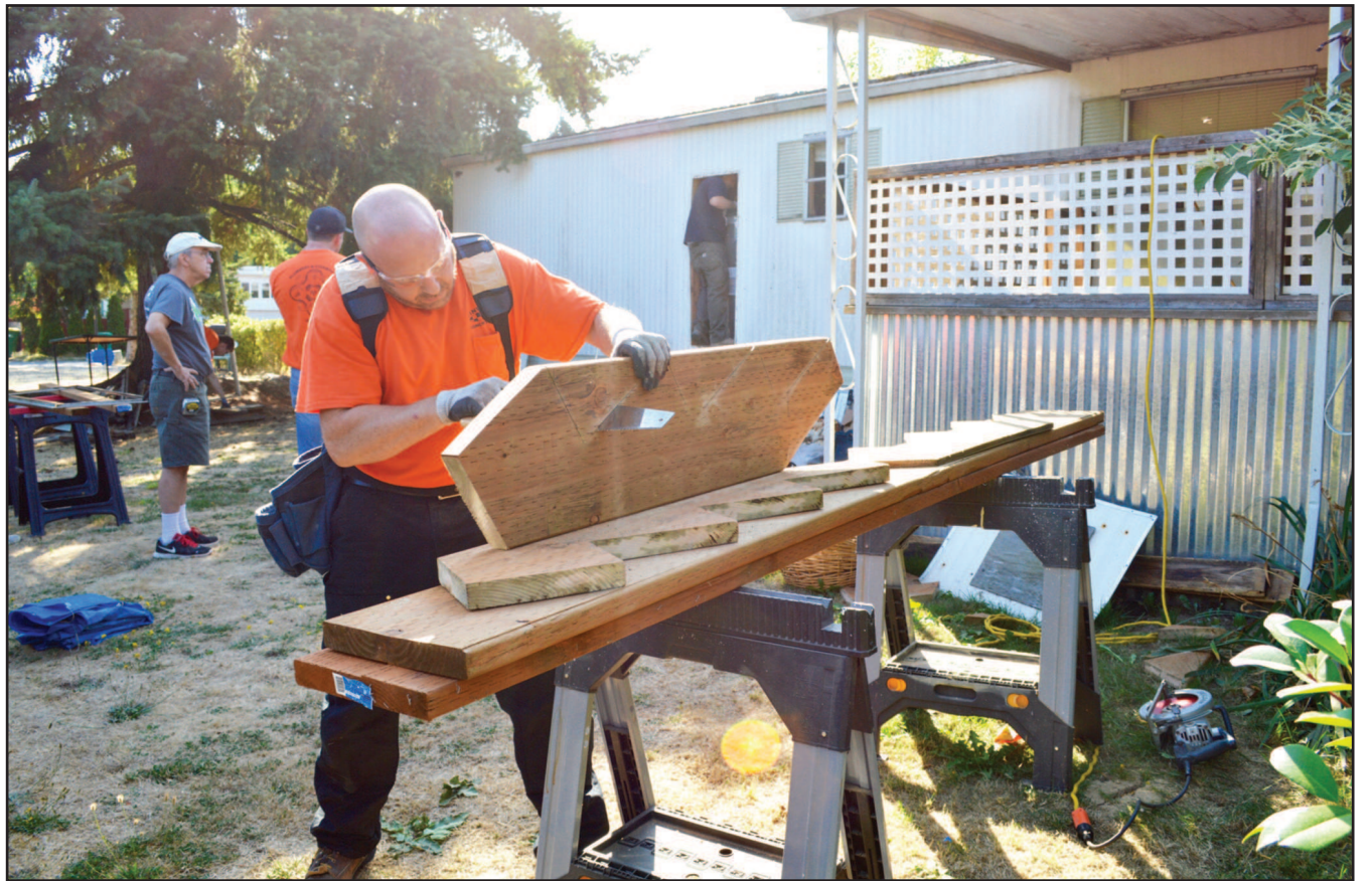
Eric "Sonny" McMahon of Laborers Local 737 cuts notches in a stair stringer. Unsafe stairs were replaced on two decks.
