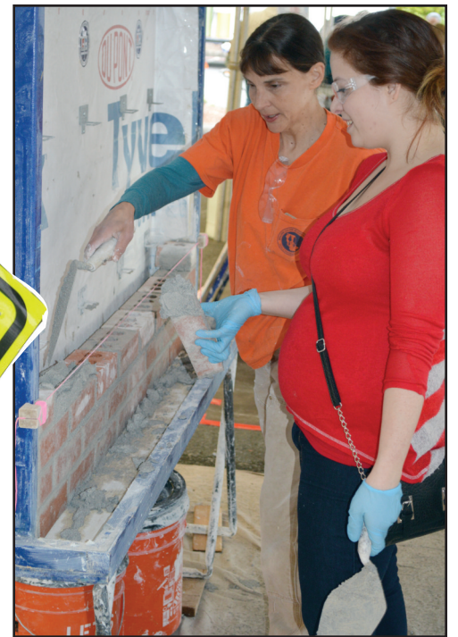
Brenda Cartino, (left) demonstrates how to butter and place a brick. The former Marine is a 12-year member of Portland Bricklayers Local 1 and a graduate of their apprenticeship program. "It's been a dream of mine since I was a kid," said Cartino. "It's a great trade. I love what I do."
