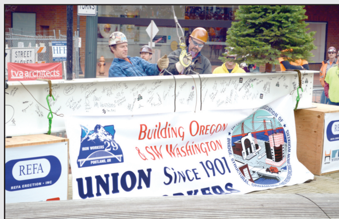
Local 29 ironworkers James Marble and Doug Green attach the final steel beam to a cable from a tower crane operated by Anson Barrow of Operating Engineers Local 701.
