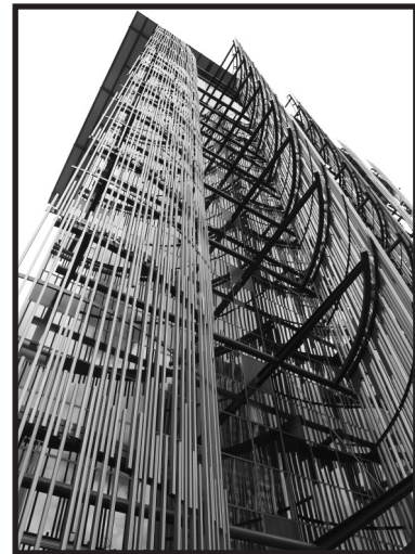
With the help of union labor, Portland's 18-story, city-block-sized federal building got a "green" remodel, and reopened in September. The names of all the workers are printed on glass at the building's entrance.
