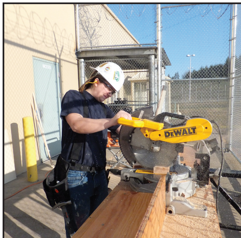
Valayshea Shaffer operates a power saw in a fenced-in area set up for an experimental inmate building trades pre-apprenticeship program. (Photo by Dave Conway, courtesy of Oregon Corrections Enterprises)
