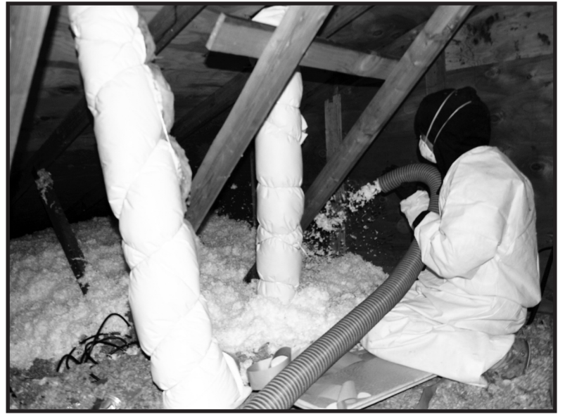
Rochelle Sadler, a member of Laborers Local 296, blows insulation in the attic of a 1986 home in Portland’s St. Johns neighborhood. She is one of 10 full-time employees at Abacus Energy Solutions. The homeowners — Oregon AFSCME lobbyist Eva Rippetateau and her husband, AFSCME international field coordinator Andy Chavira — chose Abacus because it’s a union shop. Chavira said $4,500 of blown fiberglass attic insulation, air sealing, and HVAC improvements will cut their energy bill — and make a couple of chilly rooms more comfortable.
