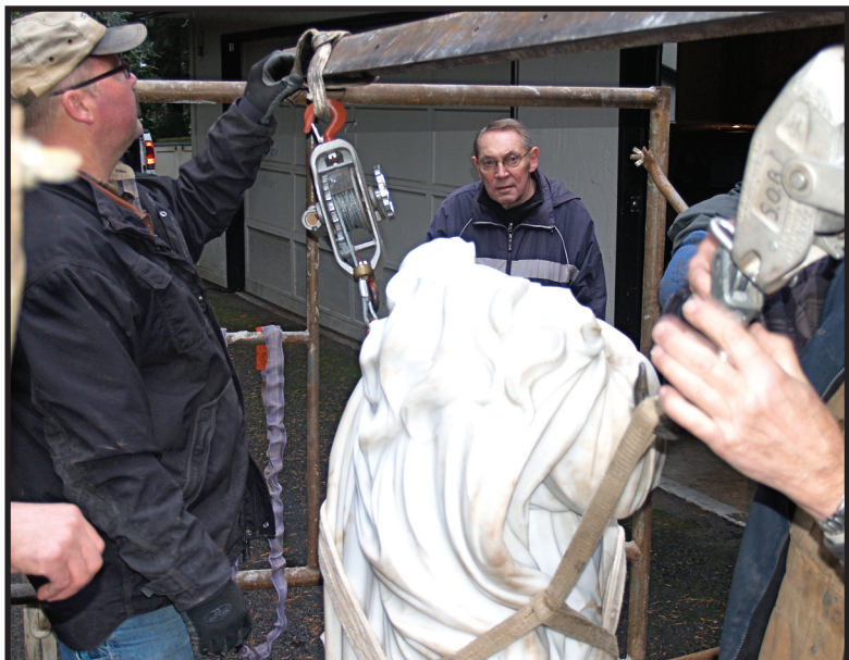
Father Jack Topper (center), executive director of The Grotto, watches closely as Mark Roddy and Steve Mahoney prepare to move the damaged statue of the virgin Mary. Mahoney is a member of Iron Workers Local 29 and Roddy is a member of Bricklayers Local 1.
