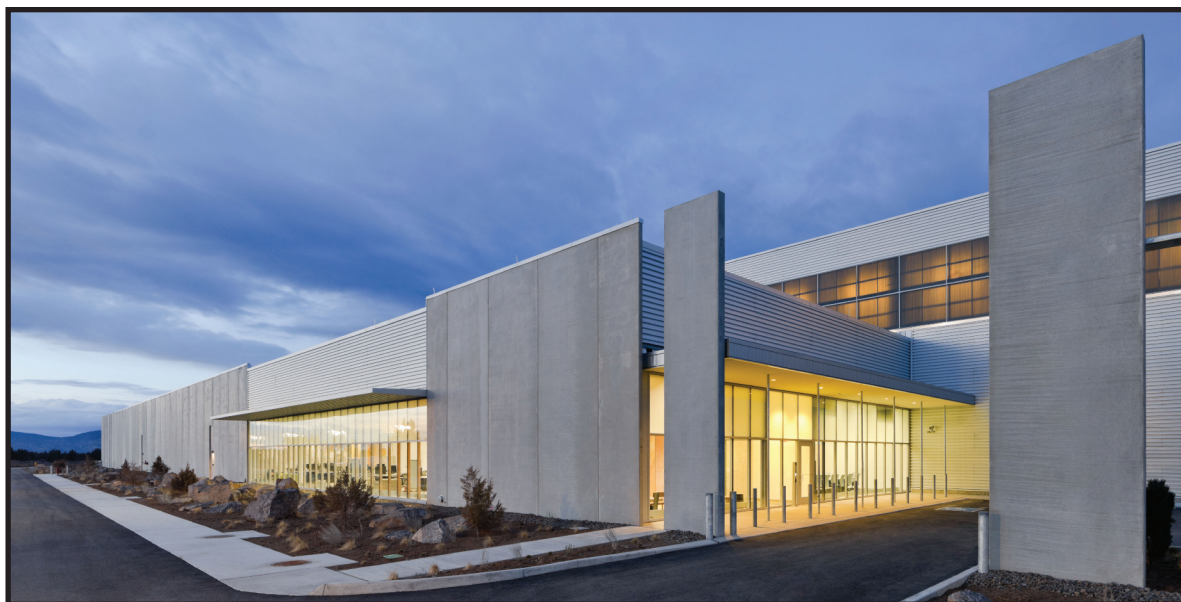
This 330,000 square foot, union-built Facebook data center is located in Central Oregon's Prineville. Data center construction is booming in Central Oregon, creating hundreds of good-paying union jobs. (Photo by Alan Brandt)
