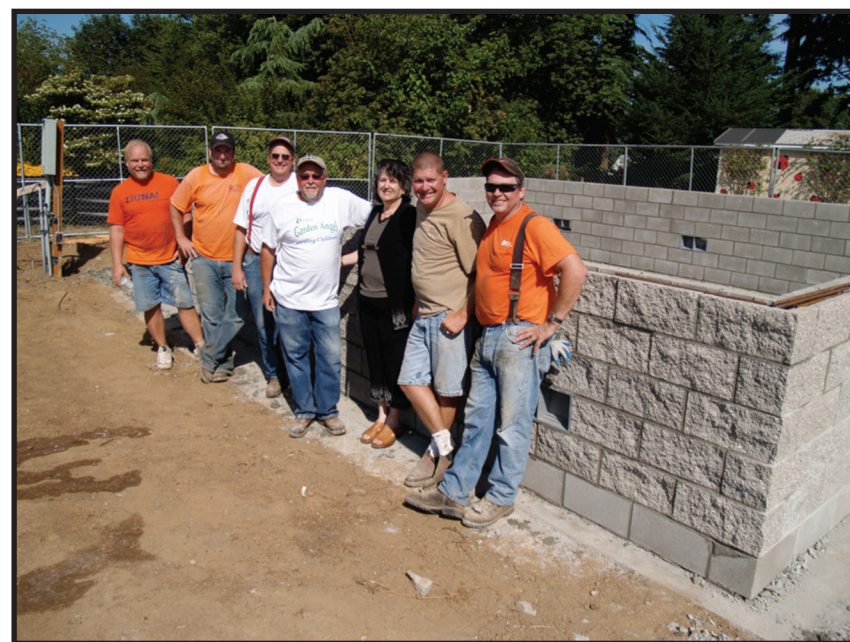
Volunteering to build a foundation for a Healing Garden greenhouse at Parry Center for Children in Southeast Portland are from left: Bill Hoffmann of Laborers Local 296, and Bricklayers and Allied Craftworkers Local 1 members Matt Eleazer, Keith Wright, Dennis Price, Shawn Lenczowski, and Scott Lummus. Standing third from right is Fran Warren, chairwoman of the Parry Center's Metropolitan Auxiliary Club.
