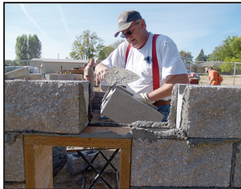
Local 1 Business Manager Keith Wright butters a block with mortar.
