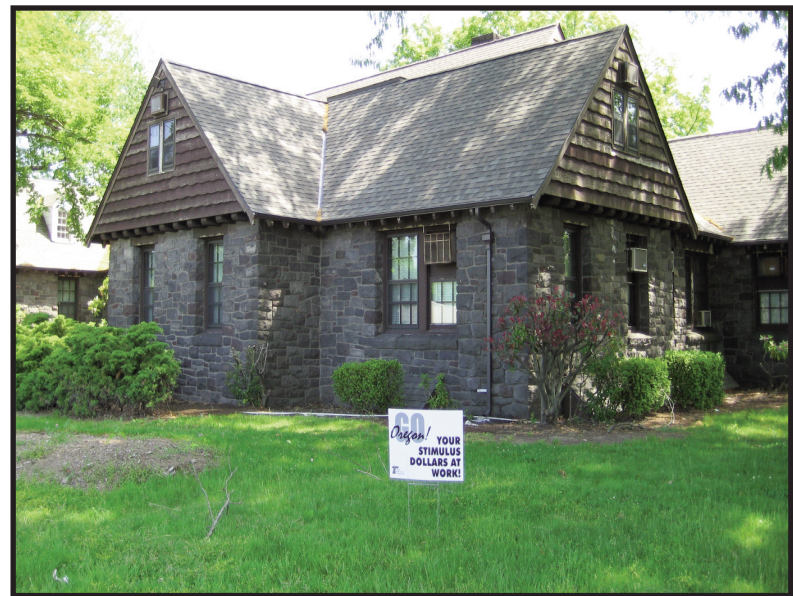
Echoes of an earlier stimulus: The stone building above, on Southeast Milwaukie Avenue, belongs to the Oregon Department of Transportation. It was built by the federal Public Works Administration, a 1930s job creation program, and re-roofed this year with funds from Go Oregon, a bond-funded $175 million state-level stimulus effort.
