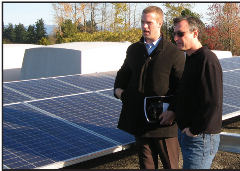
SunEdison program manager Jeremy Barnett (left) walks Multnomah County Commissioner Jeff Cogen through a photovoltaic array installed on the roof of the Yeon maintenance building. Because of the way the deal is structured, the $7 million-plus project is not subject to requirement to pay the prevailing wage. Photo courtesy of Multnomah County Commission
