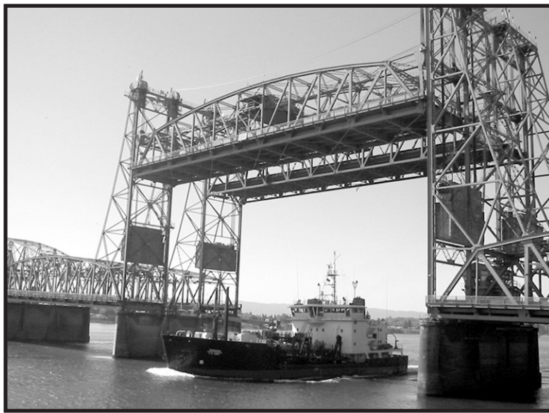
The Interstate 5 Bridge between Portland and Vancouver is actually two bridges right next to each other. One carries northbound traffic and the other carries southbound, with three lanes in each direction. There is a vertical lift in the bridge to allow boat traffic to pass.
