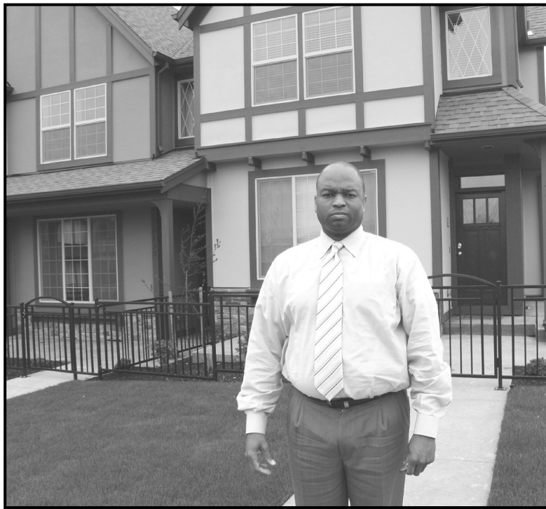
Willie Higgins is one of a dozen early homebuyers at the new Arbor Parc Bethany development in Beaverton. For over a month, he and the others had to drive five miles to pick up their mail because of a USPS decision to privatize mail delivery.
