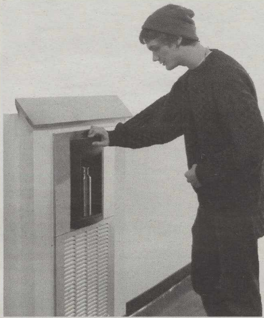
Photo by Austin Cummins Scott Senkel, senior, uses one of the recently installed water bottle filling stations to fill up his water bottle. While the filling stations have helped the school become more eco-friendly, they don't help students if students don't have bottles to fill.
