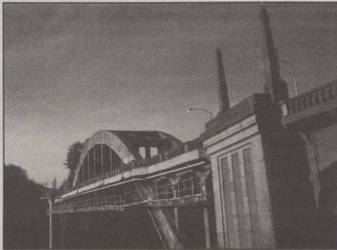
In 2010, the Oregon City Bridge will be closed for construction. The bridge was first opened on Jan. 1, 1923 and served as a shortcut for many commuters. Construction will not be completed until 2012.
