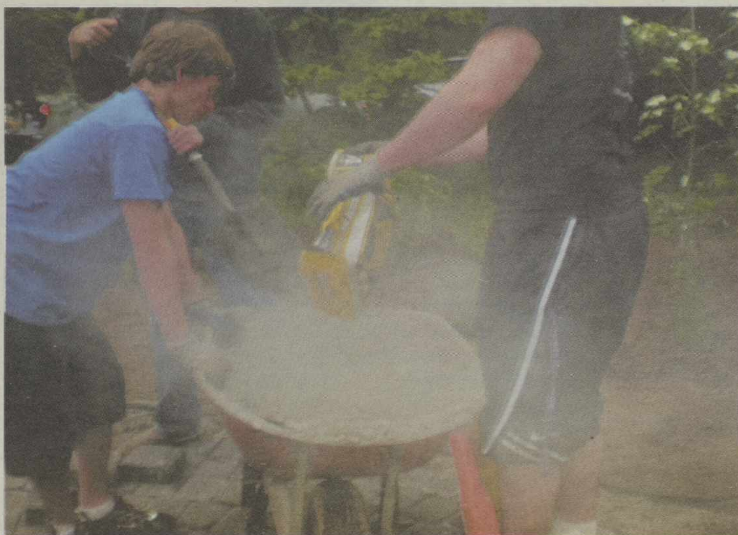
Nicolas Michels and Charles Steele mix cement for the base of the fire pit. The West Linn Parks and Recreation Department was crucial in helping the group fund and organize the service project.
