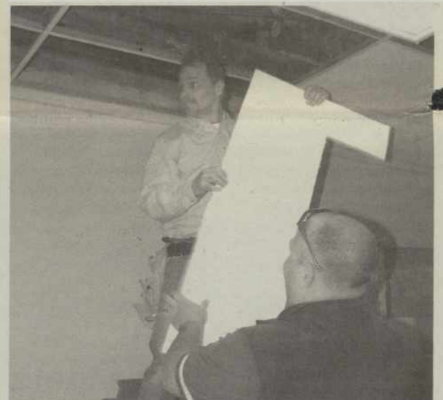
Dave Baer and Jeff Chambers, maintenance workers for the West Linn-Wilsonville School District, hang new ceiling tiles in the 700 building. Many of the old ones were infected with asbestos and had to be replaced.
