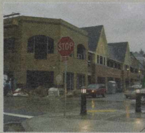
West Linn Central Village, off of Highway 43, will officially open to the public in January. The shopping development will include such businesses as Cold Stone, Quiznos and Booster Juice.
