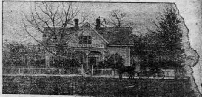
THE FOSTER RESIDENCE.
