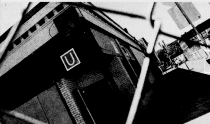
The Dirty Duck, moments before demolition
