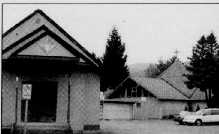
The Knights of Columbus Hall (foreground) is owned by Our Lady of Assumption Catholic Church (background) and was found in noncompliance with British Columbia's civil rights laws.
