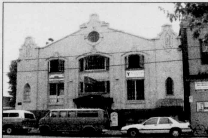
The building's gothic facade is being repainted with soft and dark browns.
