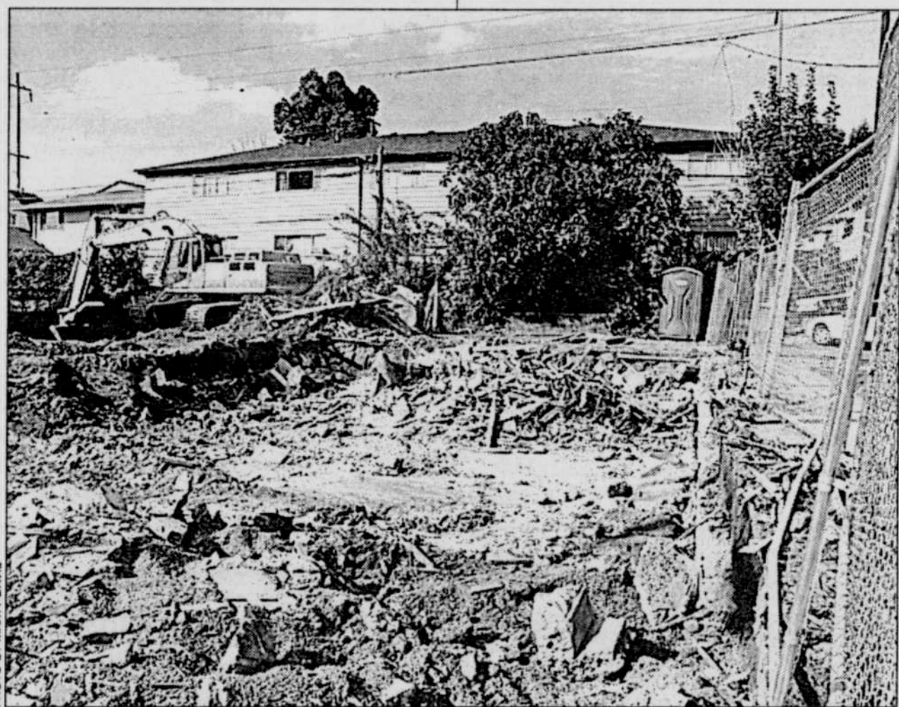
Construction is under way for the new Cadillac Cafe
