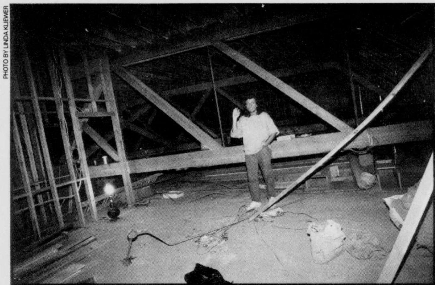
Not ready for show time: Don Horn at the future home of triangle productions! and Stark Raving Theatre Company
