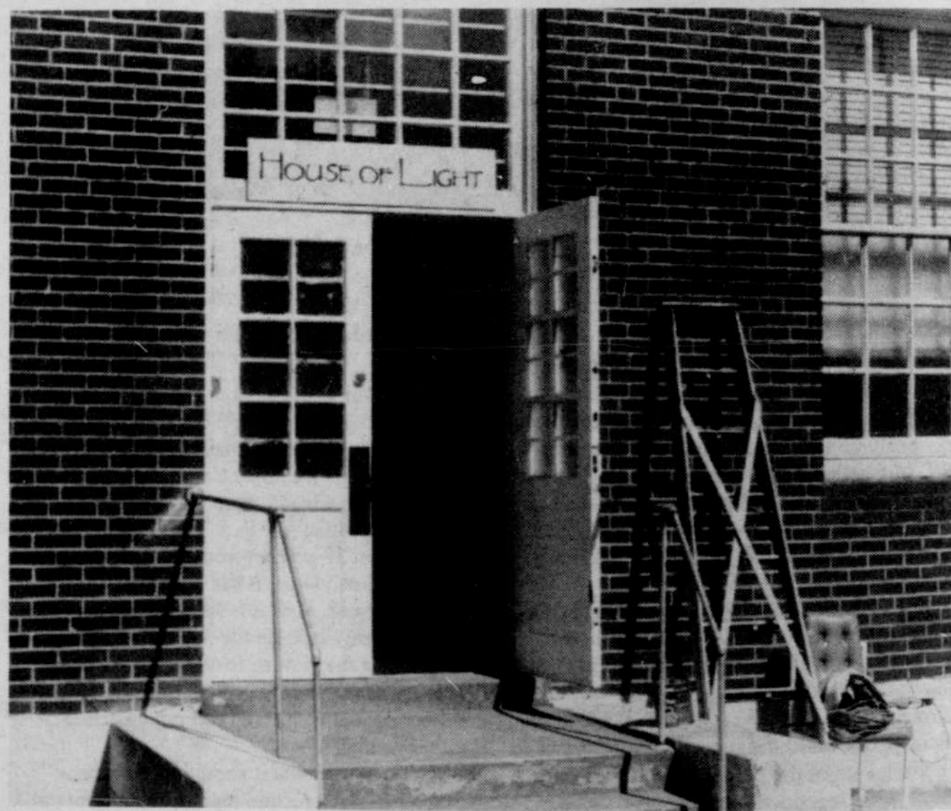
House of Light's front entry off Dekum Street in north Portland.
