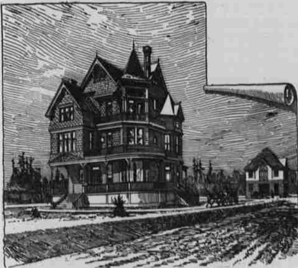
RESIDENCE OF W. M. KILLINGSWORTH, ALBINA.
