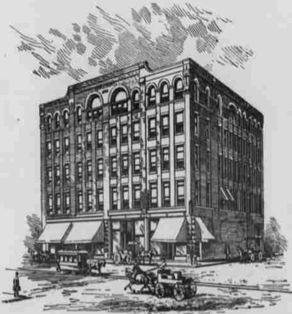
The Temple Court is one of the fine structures of Spokane Falls erected since the fire last year. It is owned by Boyd Bros. The building stands at the northwest corner of Riverside and Washington streets and its neighbors on all sides are equally imposing edifices. The cost of the Temple Court was about $70,000. Pressed brick, iron and granite enter into its construction. The ground floor is used for stores and the upper stories for offices.
